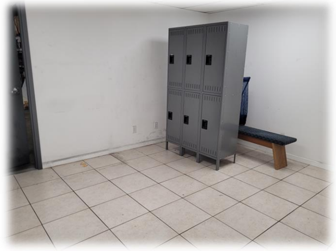
Old service area/hallway, soon to be locker room (door on left leads to shop)
