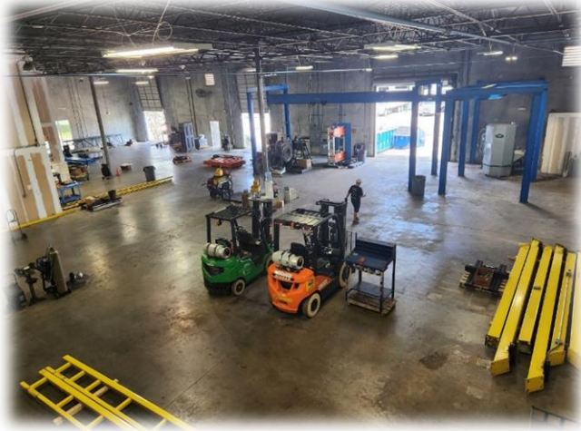
Overhead shot of the Jax warehouse showing the blue I beam crane setup in place; similar footprint will be reconstructed in Lauderdale for the test stand/paint area
