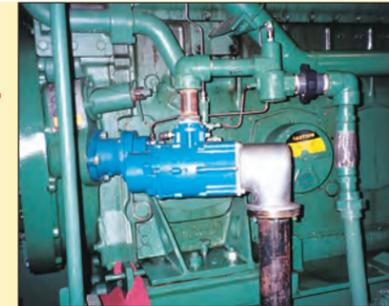
The TurboTwin Model T100-V starter's offset and overhung pinion design provides a "bolt-on fit" to most large-displacement industrial engines. It installs in minutes when replacing other turbine-type starters. (Shown here on a Cooper Superior Series 2408G Spark-Ignited Gas Engine.)
