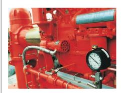
T306-I mounted on Caterpillar 3406 Engine for fire pump application
