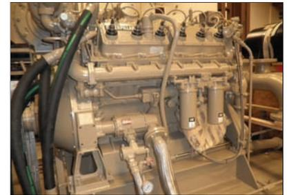
*T106-F installed on Caterpillar 3412 engine.*
