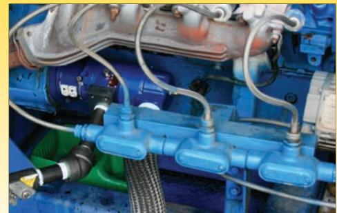
T20 installed on 5.9 Cummins engine.
