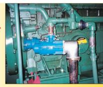
The TurboTwin Model T100-V starter's offset and overhung pinion design provides a "bolt-on fit" to most large-displacement industrial engines. It installs in minutes when replacing other turbine-type starters. (Shown here on a Cooper Superior Series 2408G Spark-Ignited Gas Engine.)
