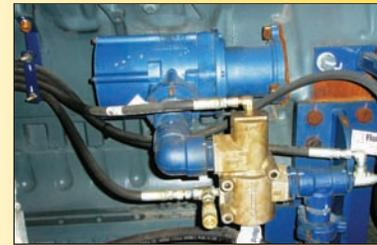
*T100-F installed on Detroit Diesel 16V2000 engine.*
