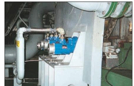
*A multiple-starter application on a Clark TCV-12 lowered air consumption by 40% over competitive turbine starters originally applied.*
